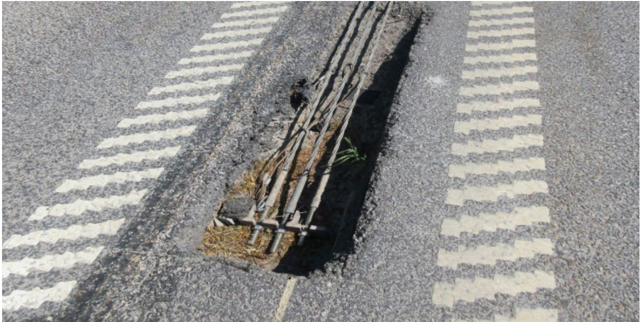
Painted rumble strip at cable terminal – Sweden (GEMS)
