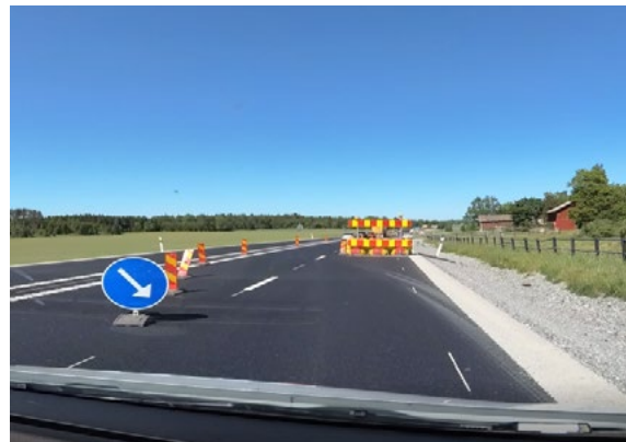
2+1 Construction Project temporary traffic control – Sweden. (GEMS)
