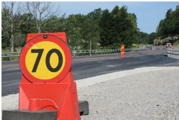
Posted speed on 2+1 construction project – Sweden (GEMS)
