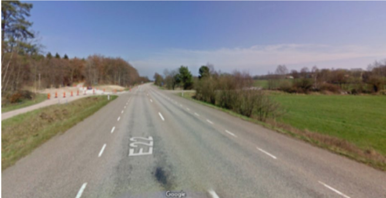
13m road platform Sweden (Google 2014)
