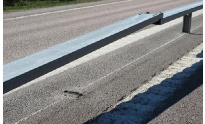
Rectangular steel lane dividing barrier (Photo - GEMS)
