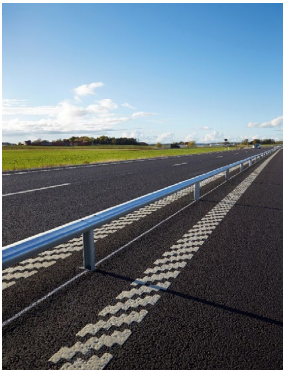
Final Installation of steel barrier (Nordic Road Safety)
