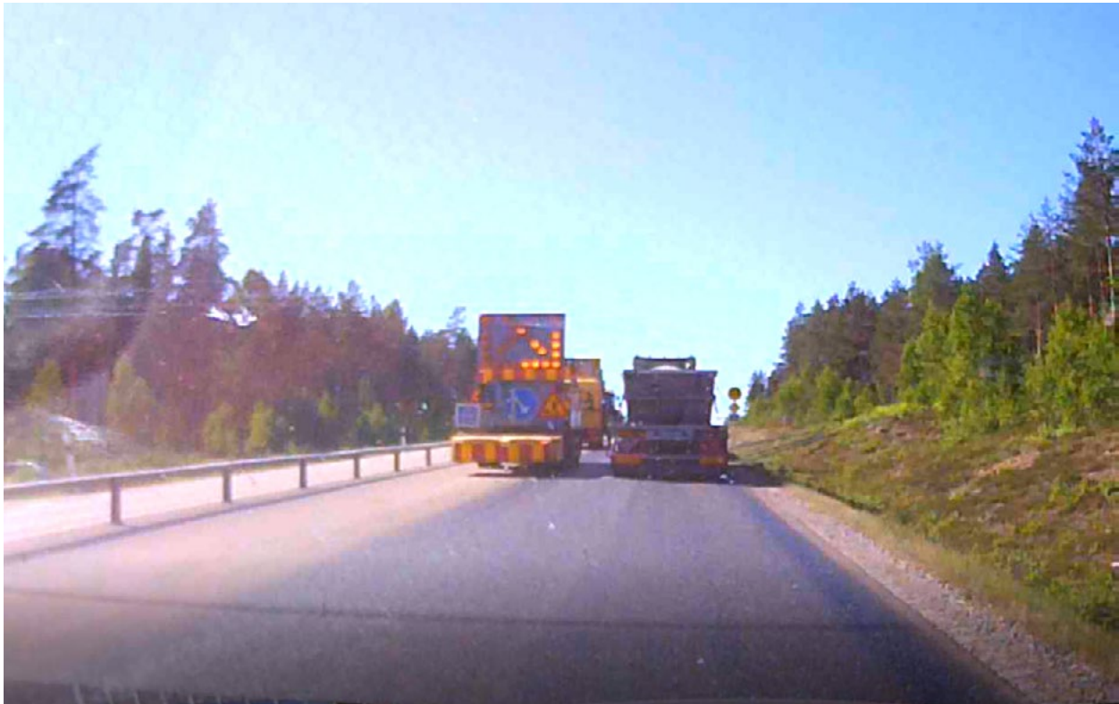
Barrier repair traffic control (GEMS)
