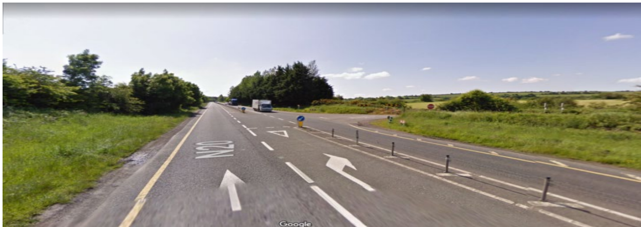
Right turn intersection – Ireland (equivalent to left turn lane in Sweden (Google)
