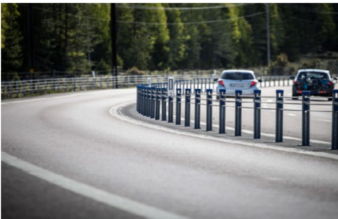
Wire rope lane dividing barrier (Photo- Trafikverket)
