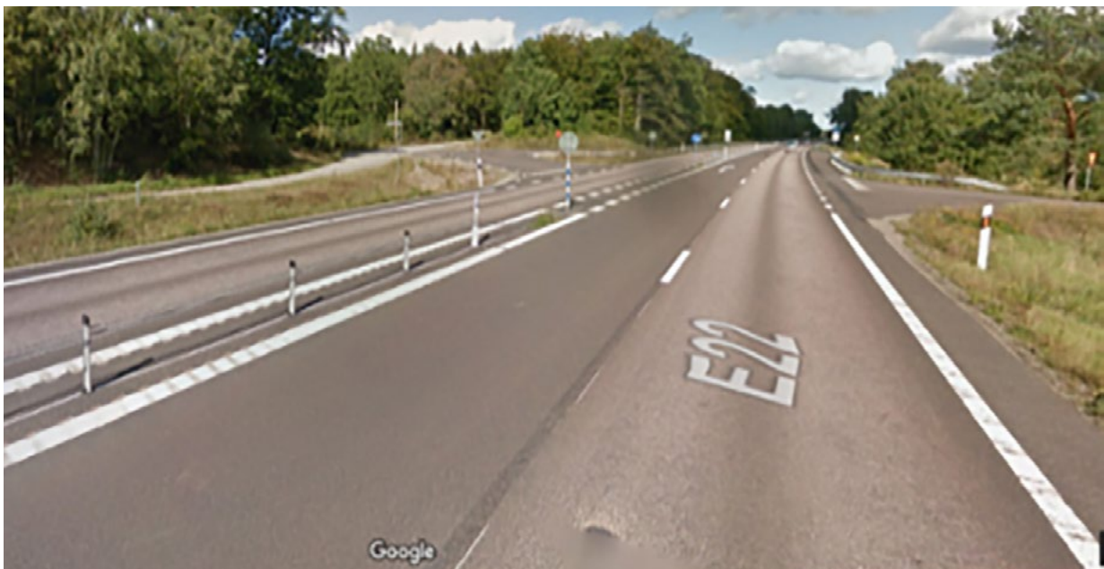
13m road converted to 2+1 – same location
