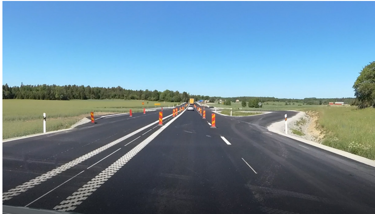
Figure 14: Construction site of a 2+1 road in Sweden
