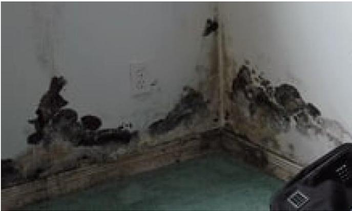
Mould in a home in Kashechewan FN after severe flooding in 2014.
